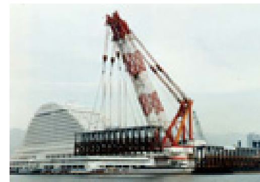
This shows the jacket being fixed in place.
