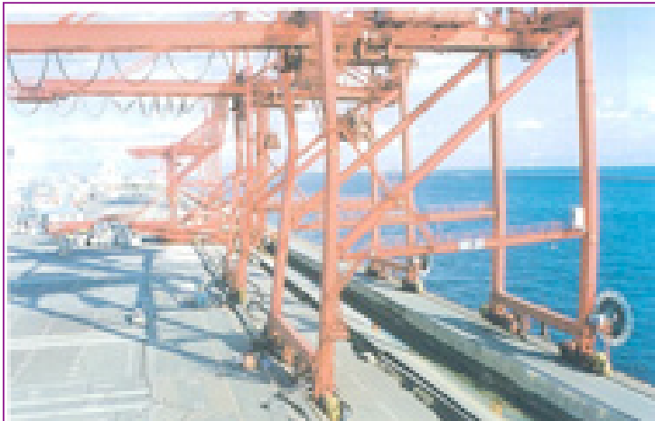
Damaged port facilities
